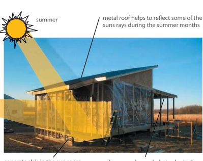
concrete slab in the sun room large overhangs help to shade the serves as a thermal mass in which building during summer months heat can be stored during the day when heat gain is not desired and released during cold nights
