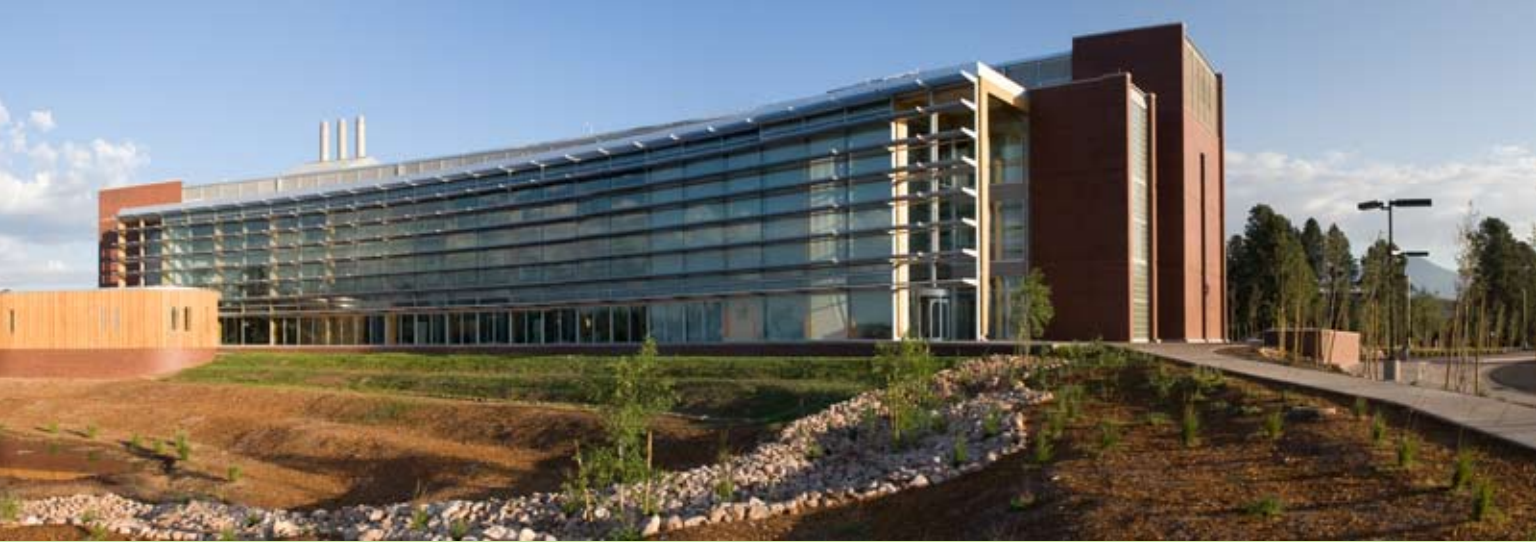
Northern Arizona University's Applied Research and Development Building received status as a LEED-certified Platinum building. It features a solar PV array, recycled denim insulation and a pervious concrete parking lot.
