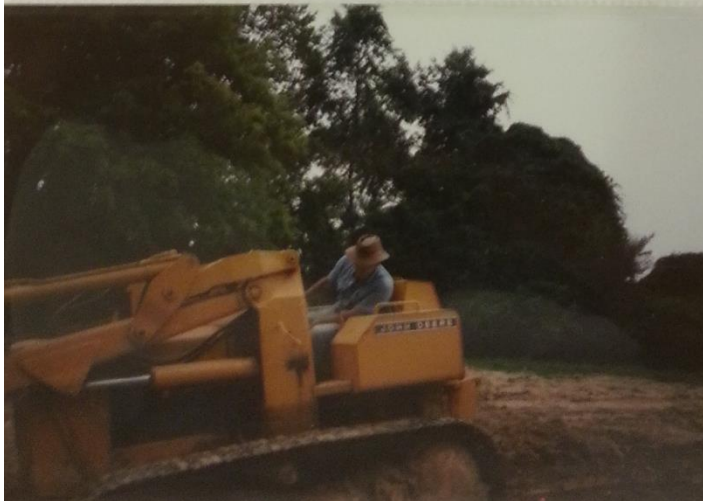
Figure 103: Clearing of the Western Enclosure Area and Possible Surface Survey Grid Establishment. Note pin flags in the central photograph. The individual pictured is R. Scammyhorn in all three photos.
