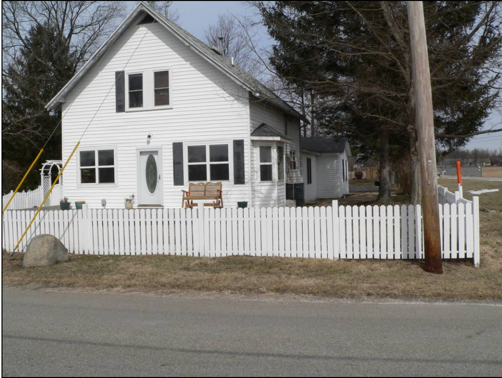
Figure 69. Site 12-Ha-358, Sugar Creek Township Schoolhouse No. 8.
