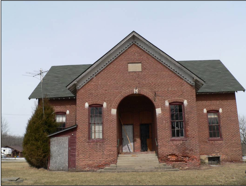
Figure 67. Site 12-Ha-356, Sugar Creek Township Schoolhouse No. 1.
