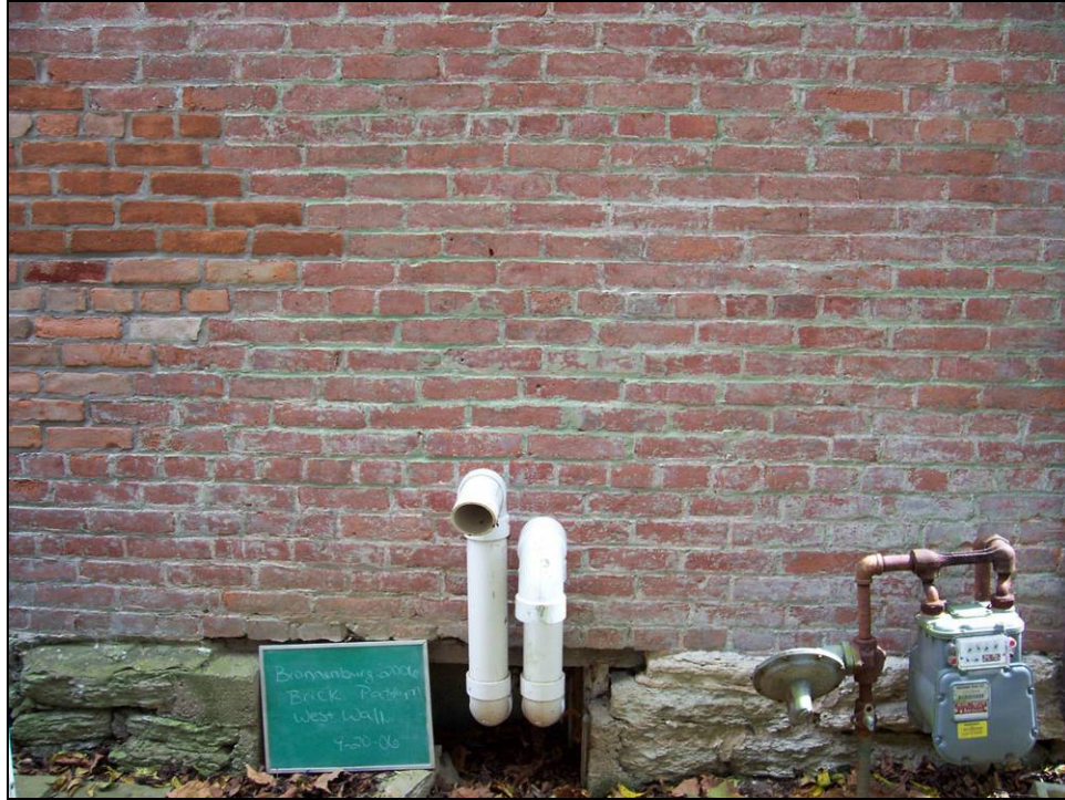
Figure 18. The American or common bond of the Bronnenberg House.
