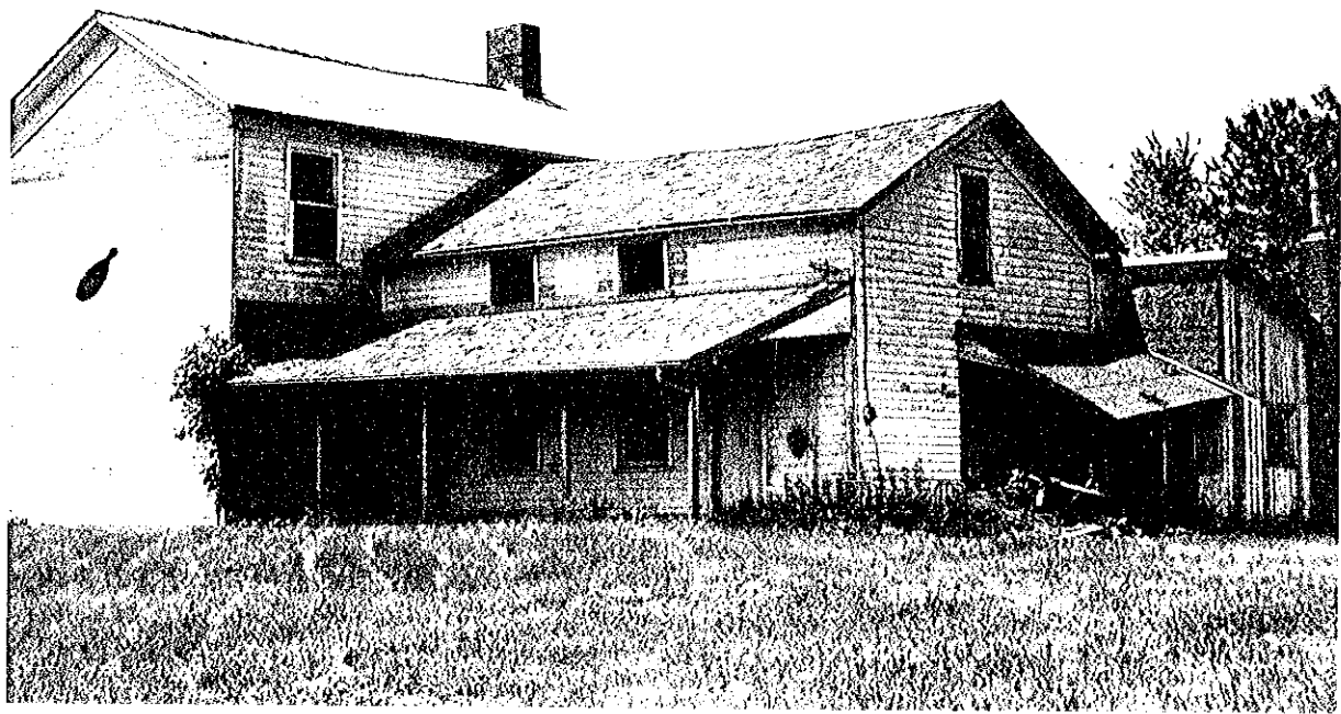
Figure 12. Looking Southwest at the East Side and Back of the House (1971) (Ball State University, College of Architecture and Planning Collection, Drawings and Documents Archive).
