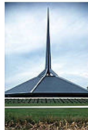
North Christian Church, Columbus, Indiana, by Eero Saarinen. Photo by David R. Hermansen
